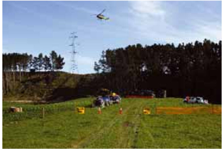
Pines close to new transmission lines were chopped out
